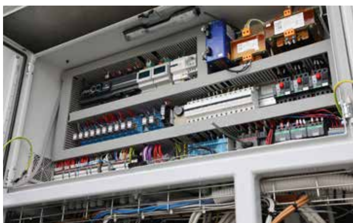
Fig. 1.d - external panel on the condensing unit with pRack and driver for ejector control
