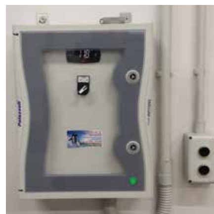
Fig. 1.c - panel on the side of the packaging cold room, with iJW controller
